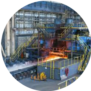
ACIÉRIES (FORGEAGE, LAMINAGE, SABLAGE)
